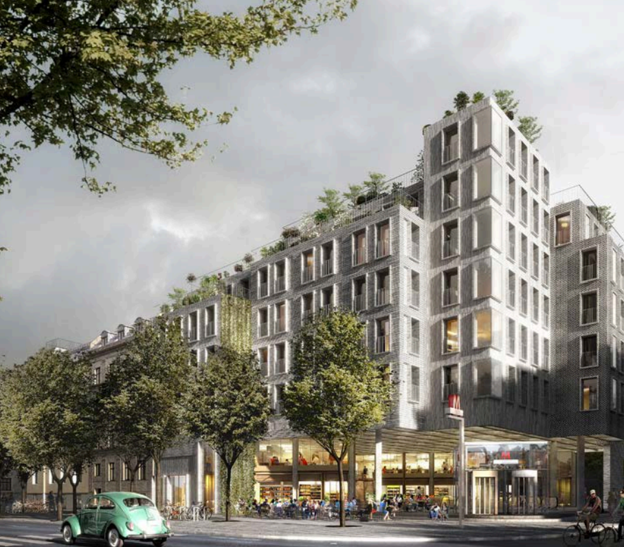
PROJECT FREDERIKSBERG ALLÉ 41, COPENHAGEN // COBE ARCHITECTS
