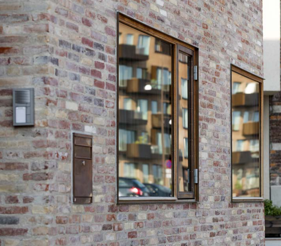
Teak windows and doors, openable sashes in copper and glass to glass corners
