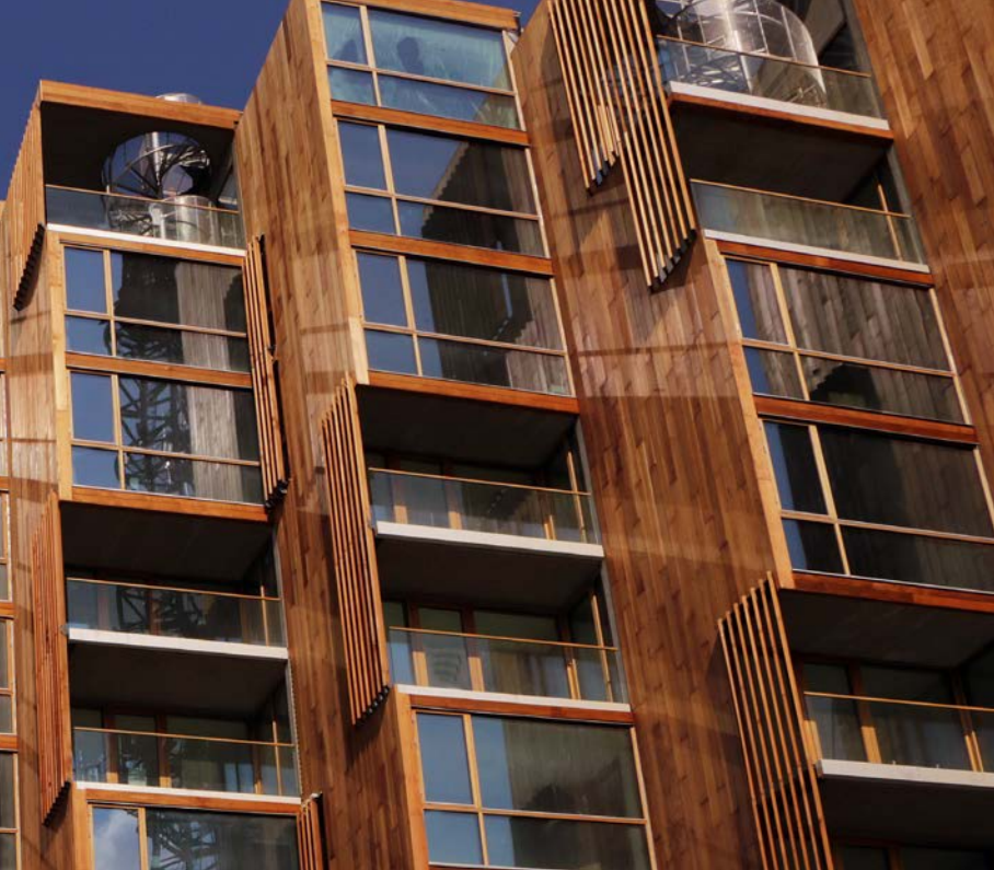
Oak windows and doors, deep frames and oak fire elements
