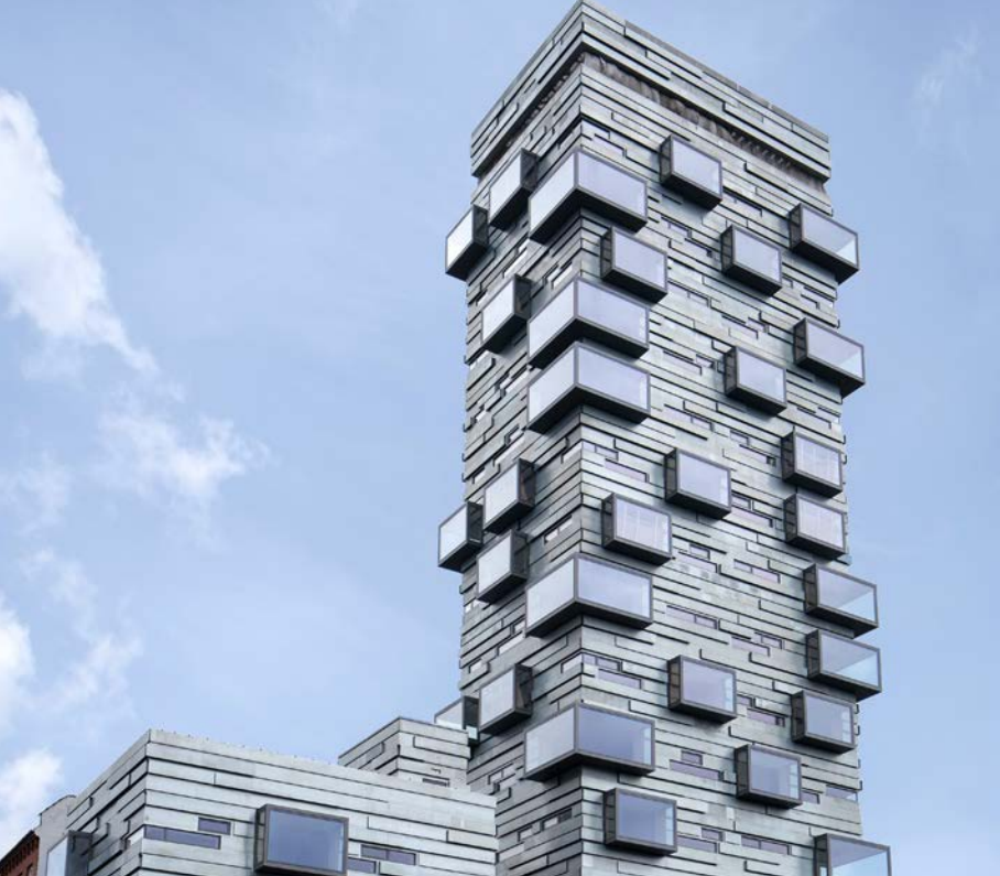
CHARLOTTETÅRNET, COPENHAGEN // LUNGAARD & TRANBERG ARCHITECTS
