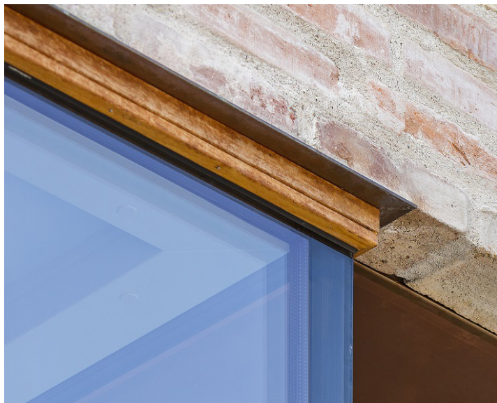
SPECIAL SOLUTION // GLASS TO GLASS CORNER
